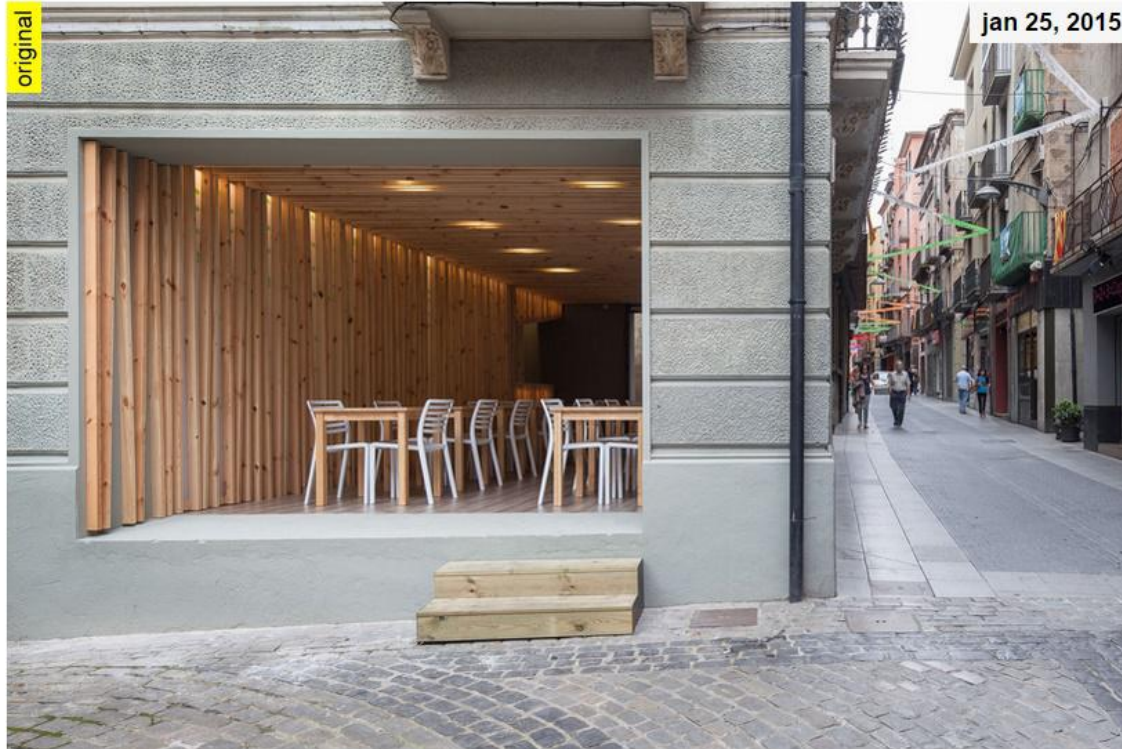
arnau estudi d'arquitectura clads spanish restaurant with timber slats
